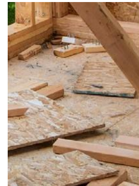
Construction board waste
