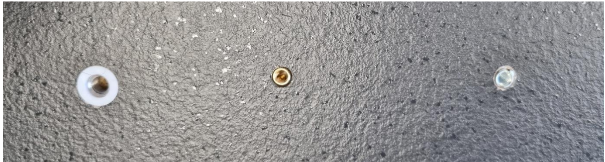
Picture 9: Couplers embedded in pre-drilled holes
