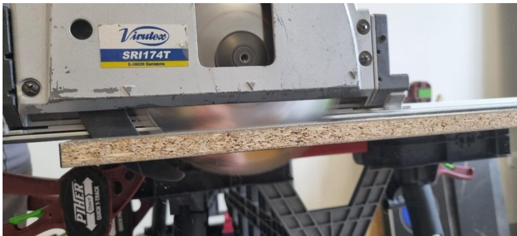
Picture 1: Sawing (cutting) the board – using a plunge saw
